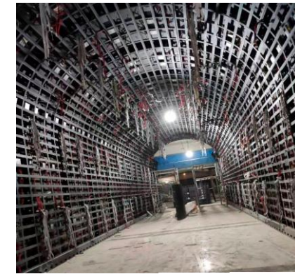
Tunnel screen structure
